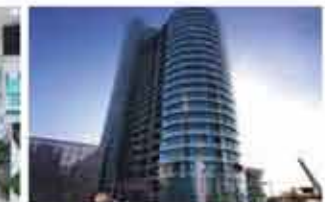
Tianjing Electric Power Company
