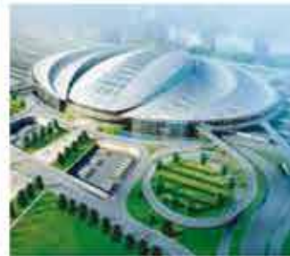
Beijing South Railway Station
